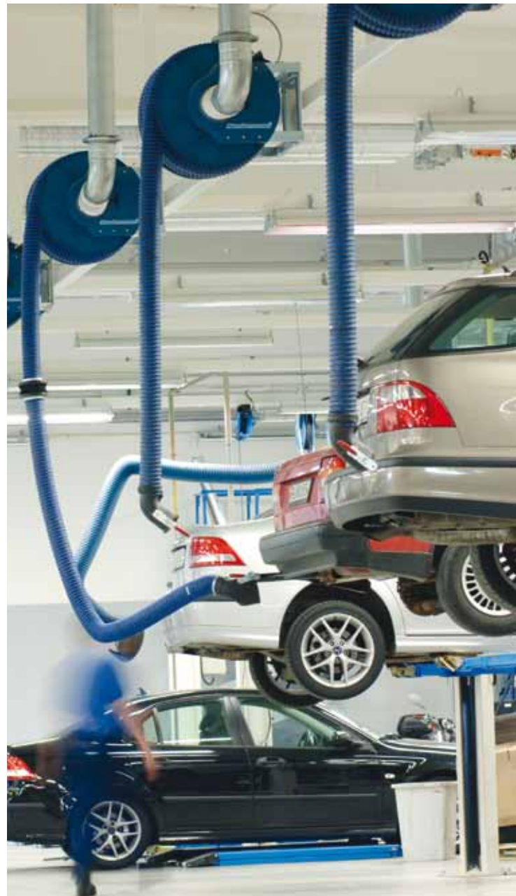
Nederman supplies a complete range of equipment for handling exhaust fumes in vehicle repair shops to ensure a clean and safe working environment.
