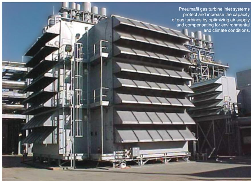
Pneumafil gas turbine inlet systems protect and increase the capacity of gas turbines by optimizing air supply and compensating for environmental and climate conditions.
