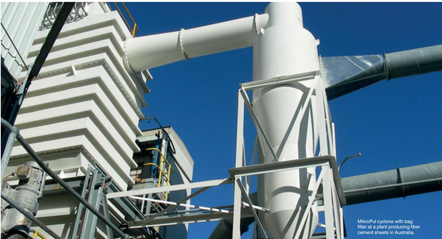
MikroPul cyclone with bag filter at a plant producing fiber cement sheets in Australia.
