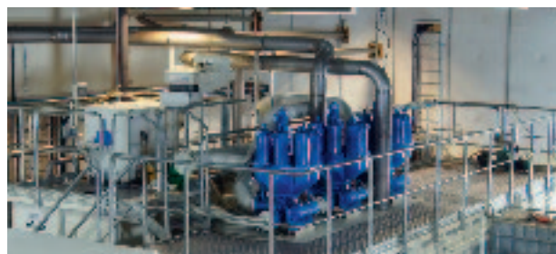
Nederman system for treatment of coolants can be applied to most machining tools.
